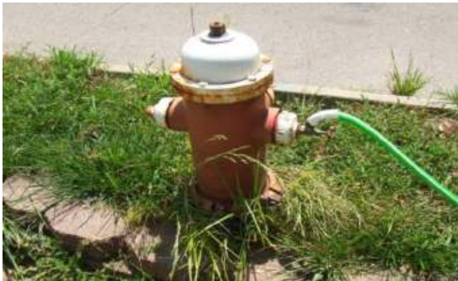
Figure 4.2. Hydrant With Un-metered and Possibly Unauthorized Use
