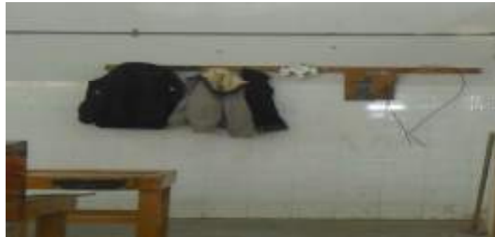
Fig. 4.6: Problem (5) in Existing Design.
