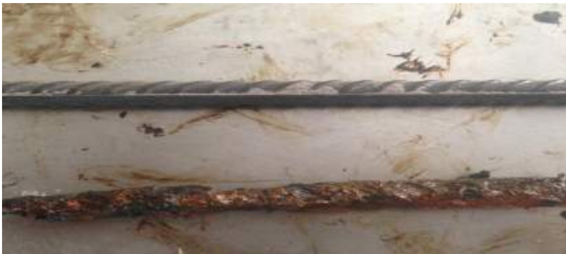
Fig 4.4: Corrosion of reinforcement in the first stage of test program.
