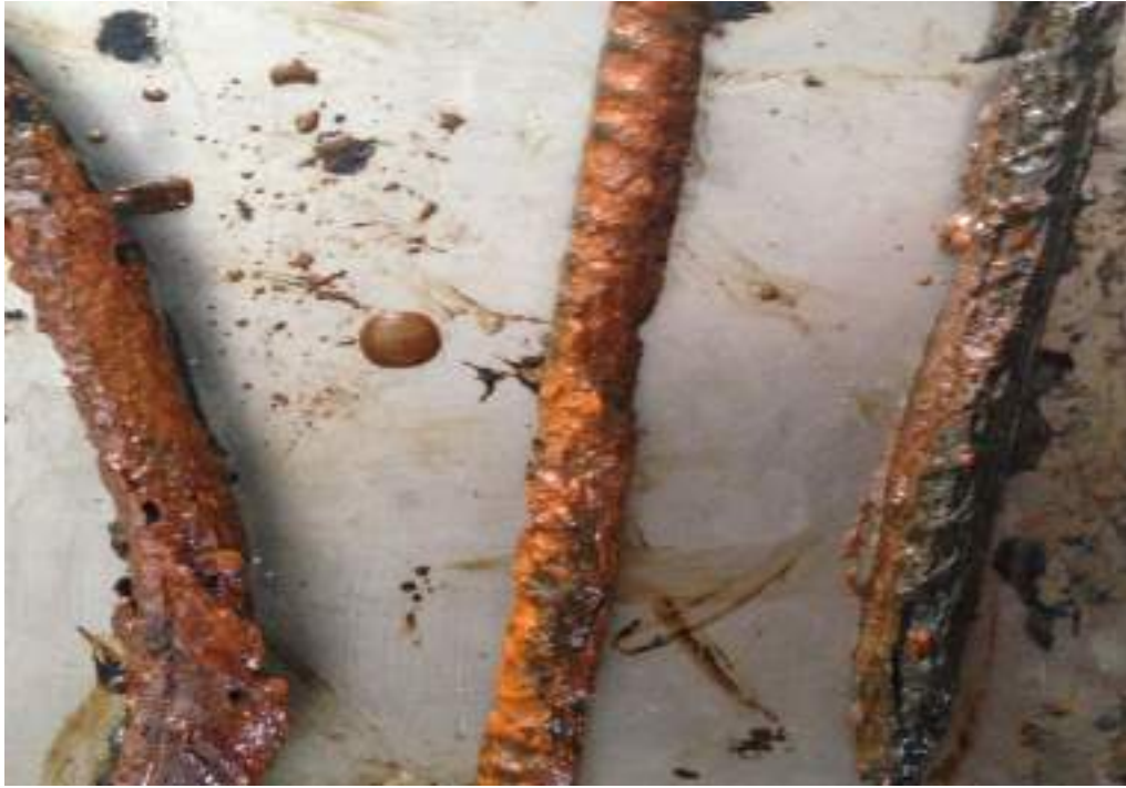
Fig 4.6: Corrosion of reinforcement in the first phase of test program.
