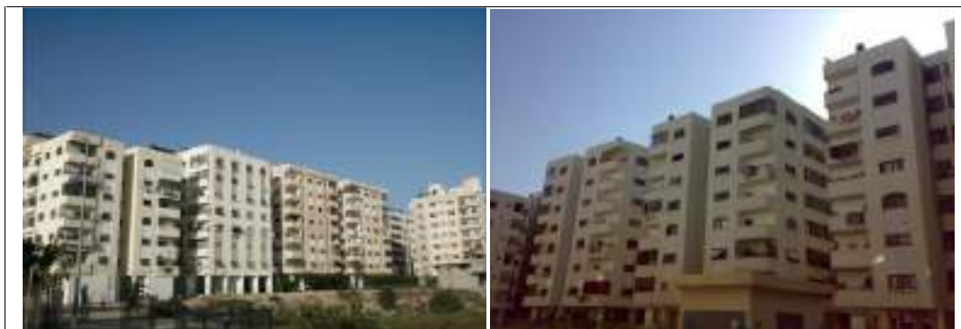
Figure (3.8): Tel al-Hawa housing project
