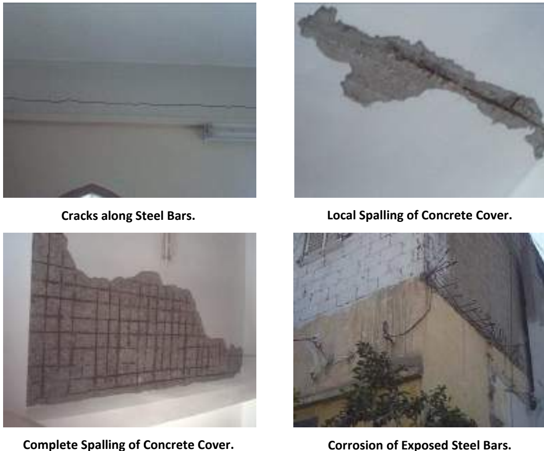
Figure 2.11: Steel Reinforcement Corrosion in Different Defects Buildings in Gaza Strip (Abu Hamam, 2008)
