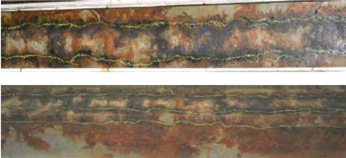
Figure 5.4: Cracks at the Bottoms Sides of Beams
