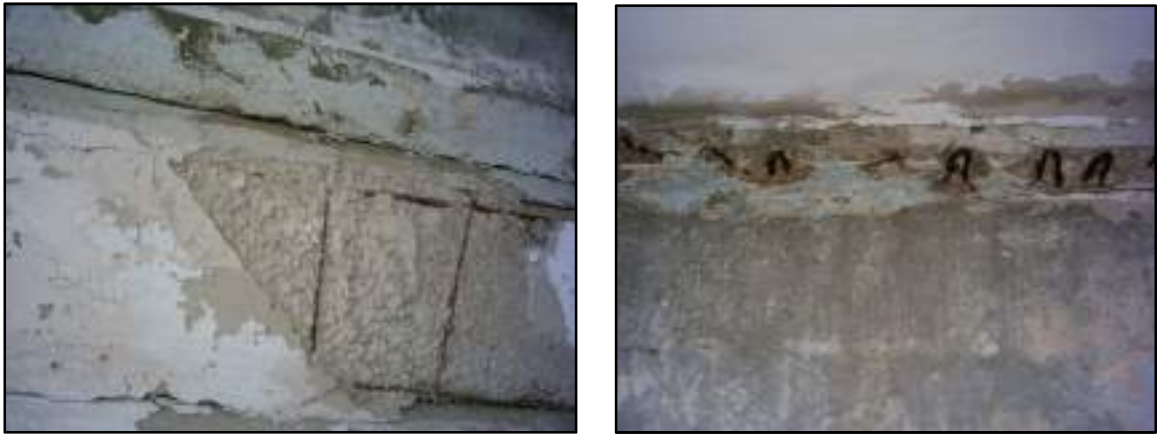
Figure 1.1: Some Pictures of Corroded Reinforced Concrete Beams
