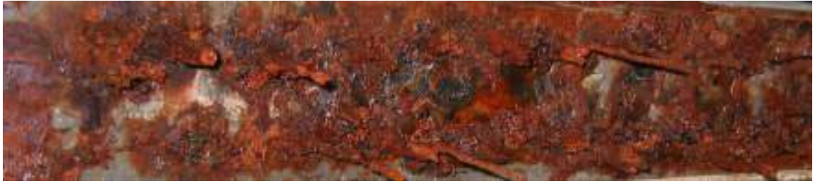
Figure 5.2: Rust on Beams during the Corrosion Process
