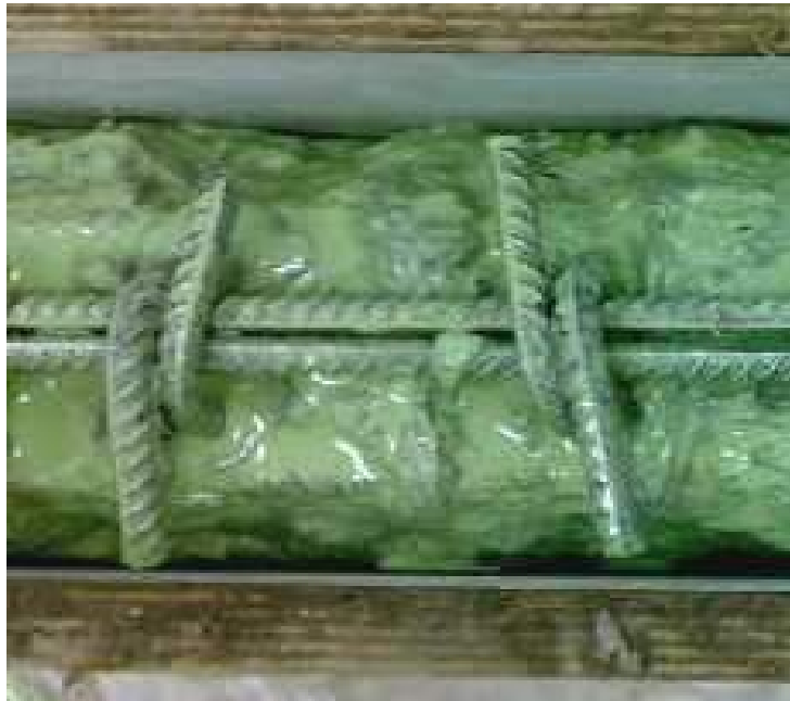
Figure 4.14: Repair Material Type 2 Brushed On Beams
