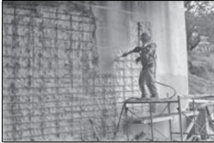
Figure 3.4: Using a Pneumatic Hammer to Remove Wall Concrete Cover (El-Reedy, 2008)
