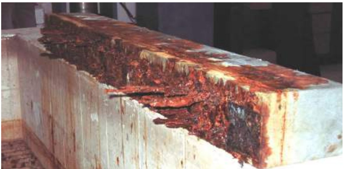
Figure 4.12: Rust on Beams at the End of Corrosion Process
