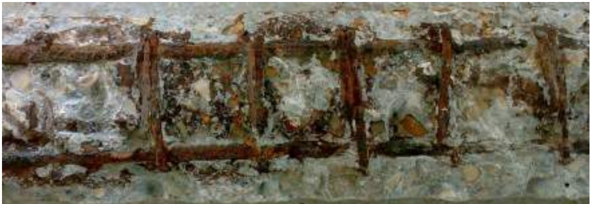
Figure 5.5: Steel Status after Corrosion
