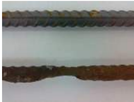
Figure 5.6: Corroded Steel Bar in Comparison with Non Corroded Steel Bar
