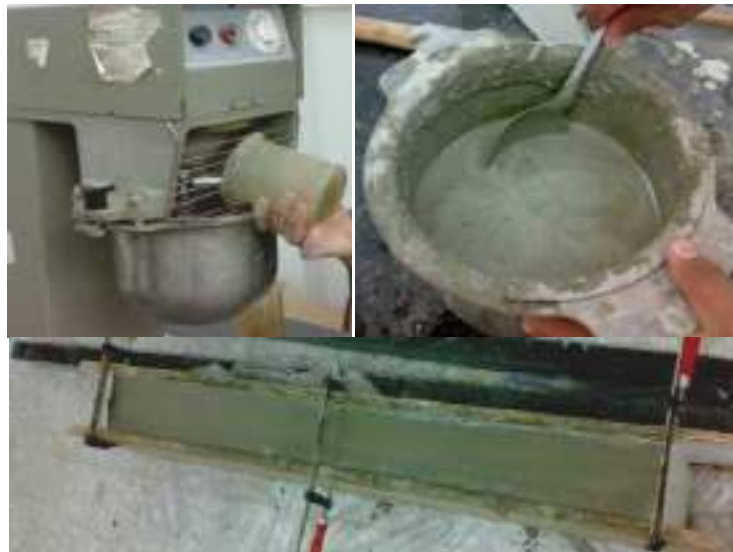
Figure 4.15: Repairing Material Type 3 While Mixing and Casting
