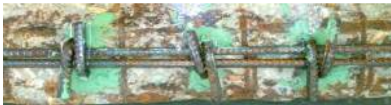
Figure 4.13: Installing Of Shear Connectors
