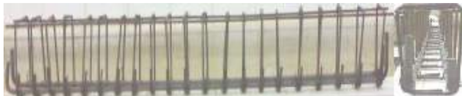
Figure 4.2: Steel Bars Cage
