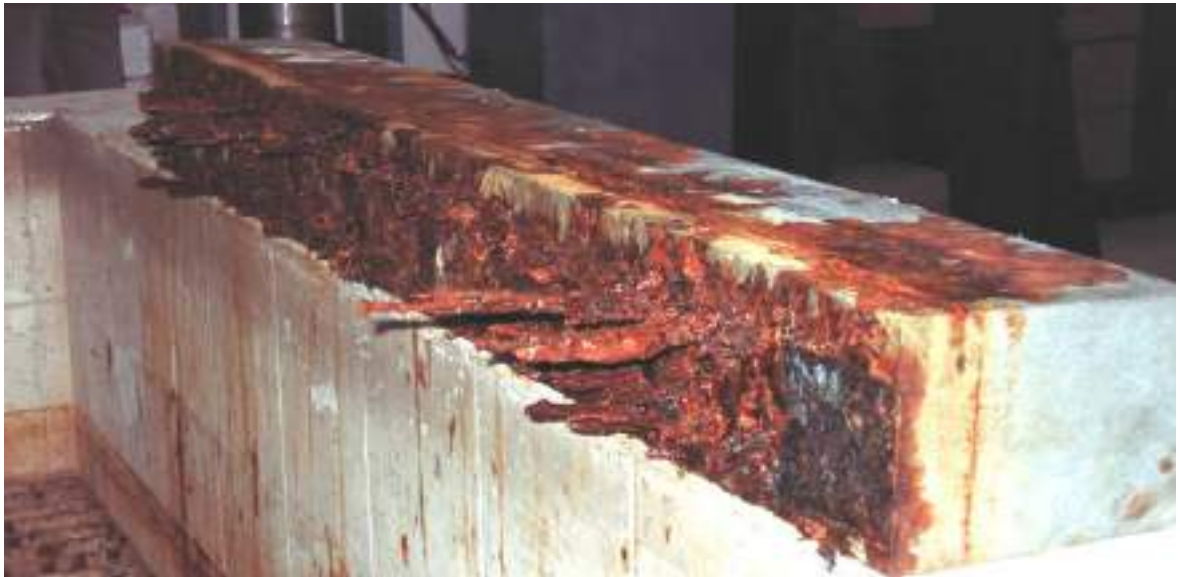
Figure 5.3: Rust on Beams At The End Of Corrosion Process
