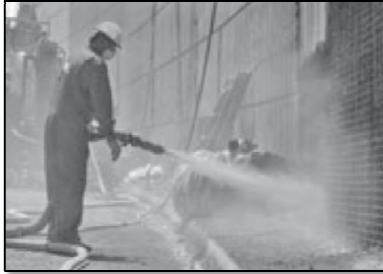
Figure 3.13: Using Shotcrete (El-Reedy, 2008)
