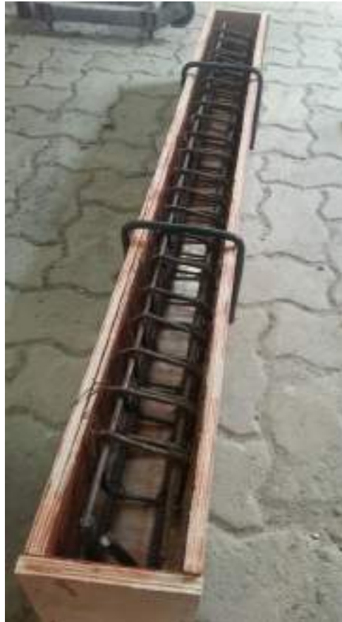
Figure 4.18 Wood form and reinforcement details
