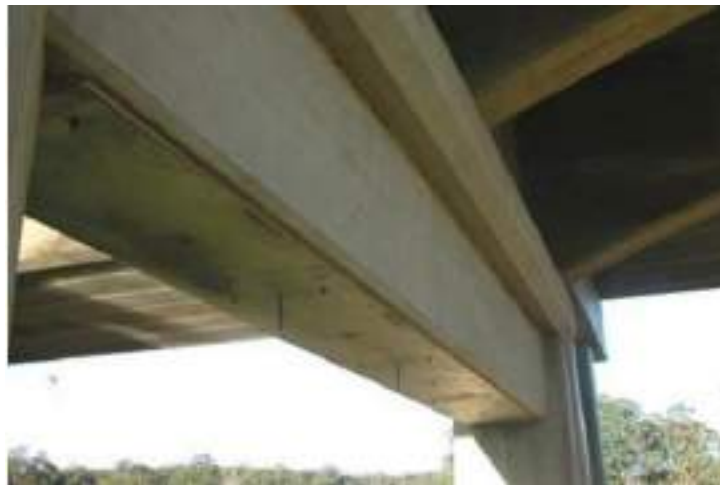
Figure 2.3 Strengthening using externally bolted steel plate (Source: Khalaf, 2015).
