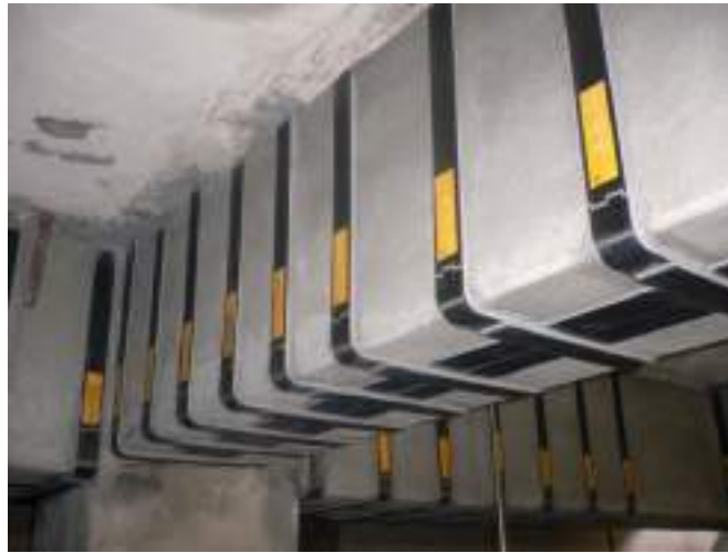
Figure 2.9 Shear Strengthening by FRP (Source: SIKA Carbodur, n.d.).
