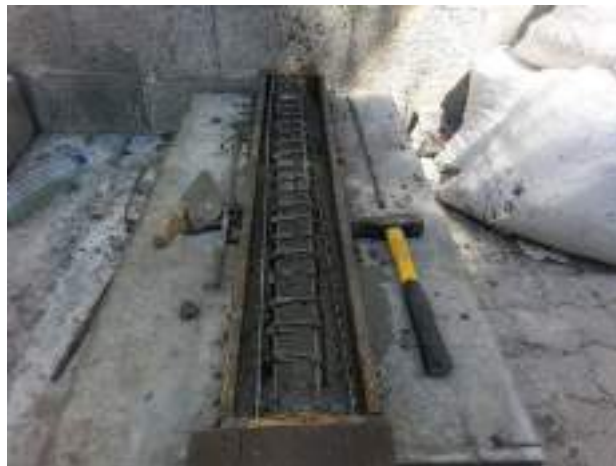
Figure 4.25 Control beam MA.B1 casting process.
