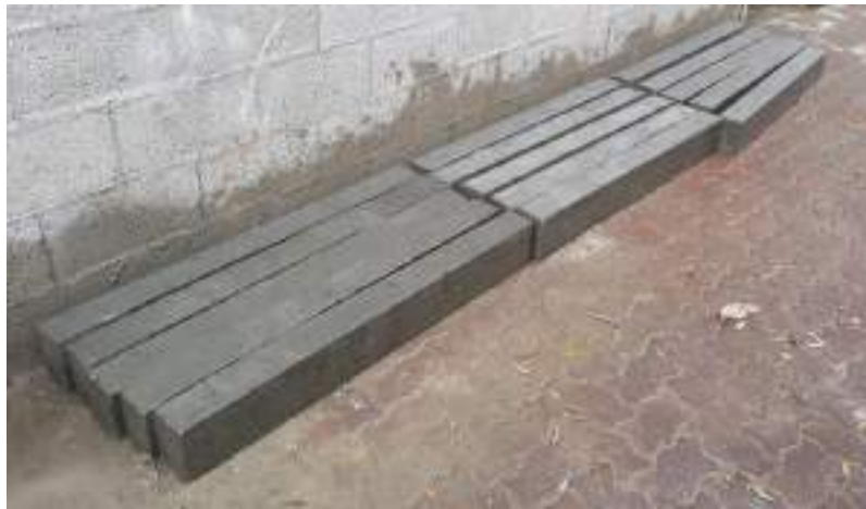
Figure 4.20 Curing process of RC beams.
