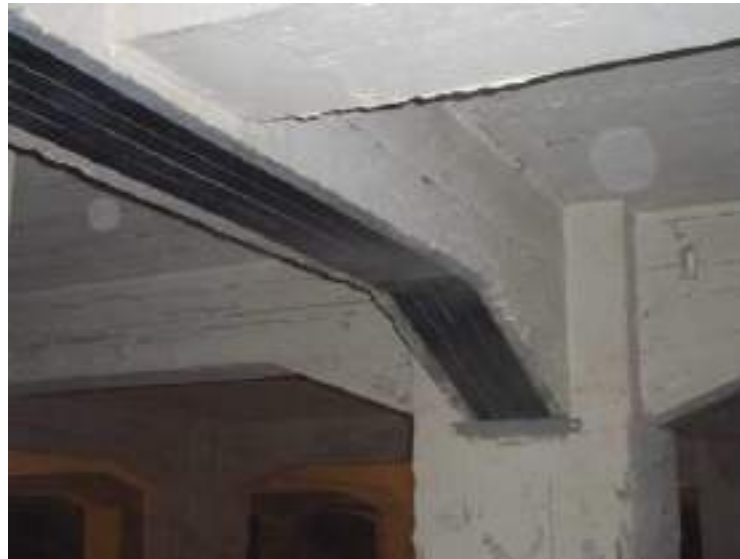
Figure 2.4 Strengthening using bonded FRP (Source: Carbon Fiber Wrapping, n.d.).
