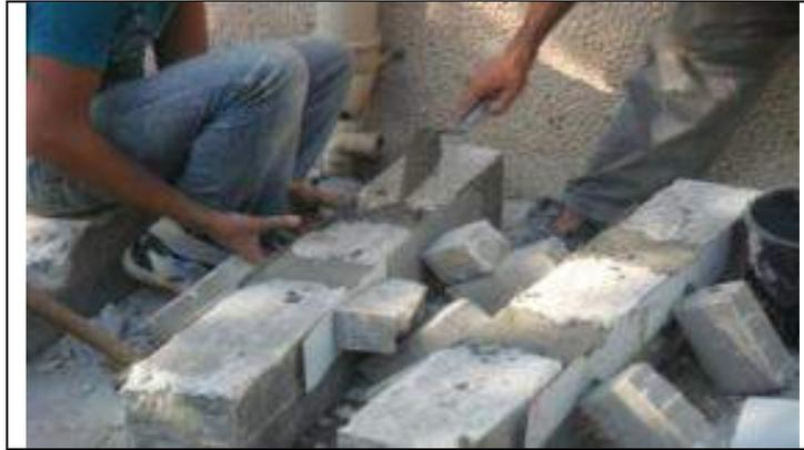
**Figure 4-6: Applying UHPC matrix to the Cracked beams**
