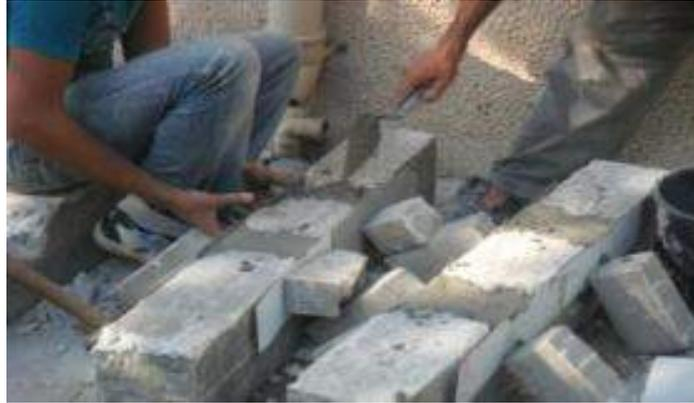
**Figure 6-7: Applying UHPC matrix to the heated beams**
