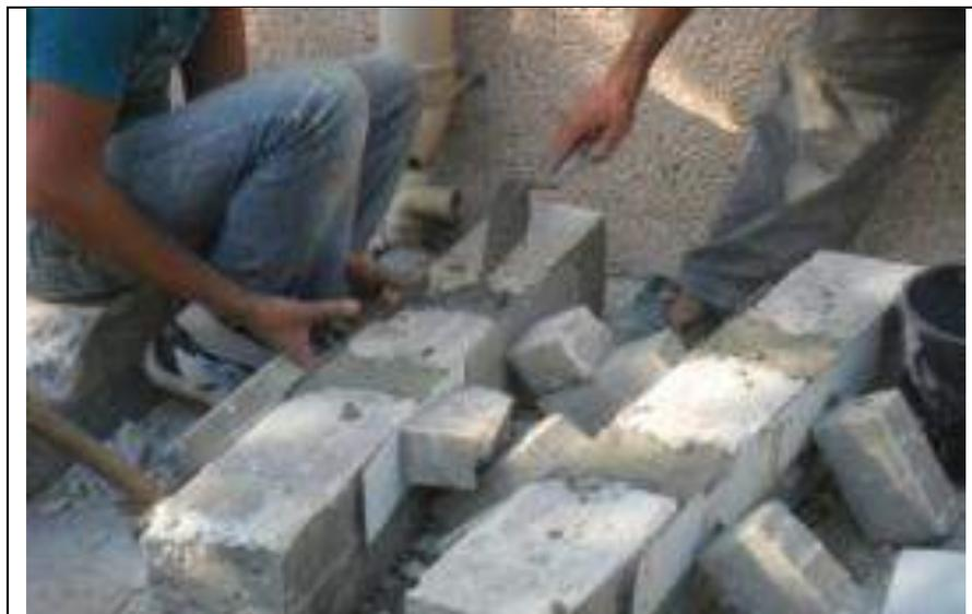
**Figure 4-15: Applying RM matrix to Cracked Beams**
