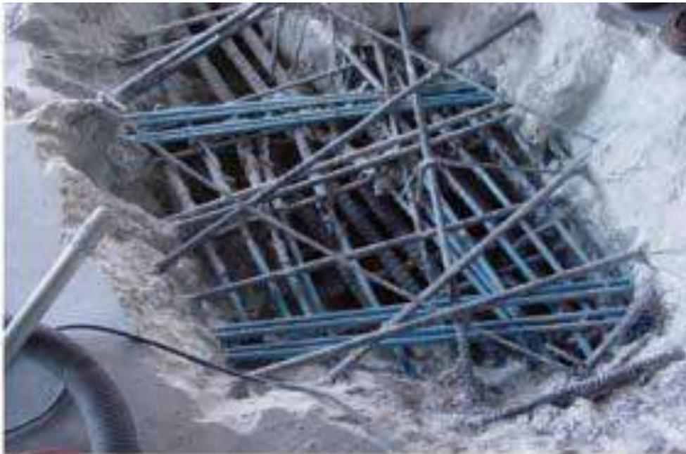
**Figure 5-1: Honeycomb in a column due to excessive lift depth**
