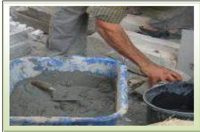
**Figure 5-10: Applying UHPFRC matrix to Honeycombed beams**
